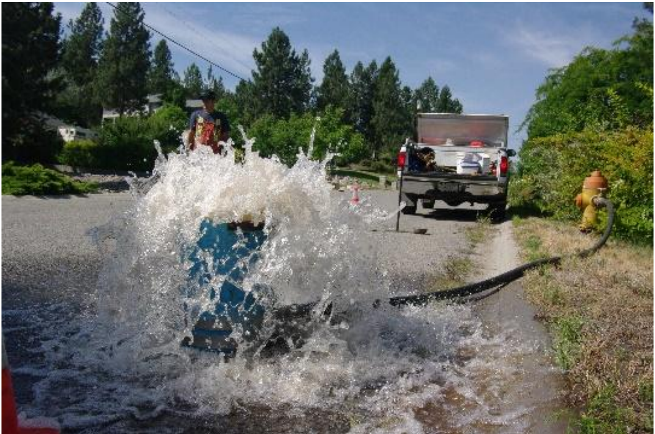
13 Flushing in Progress
